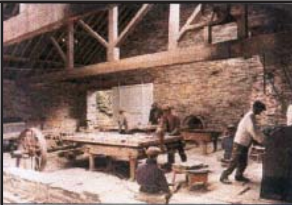
Splitting and dressing the slates in the mill.
