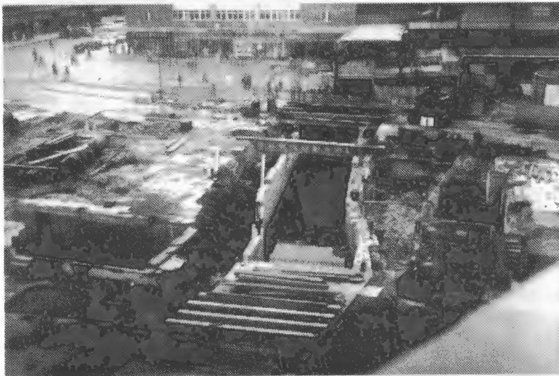
The last view of Smithford Street and culverting the River Sherbourne
