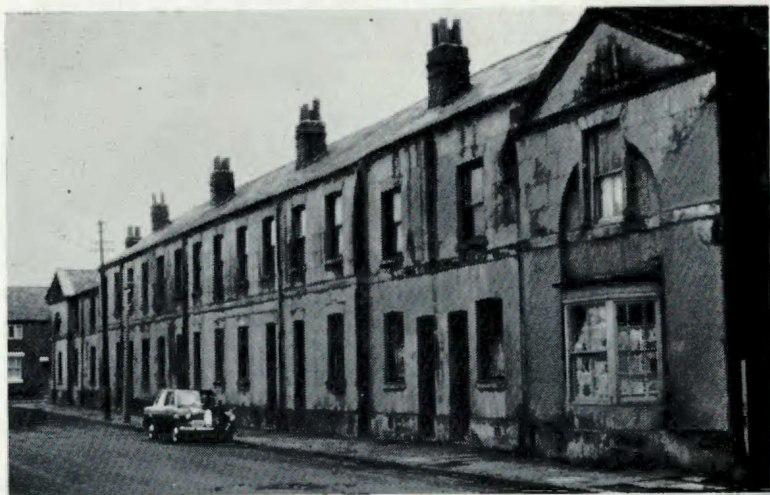
Plate XIV. Bedworth Worsted Mill in 1966, shortly before demolition.
