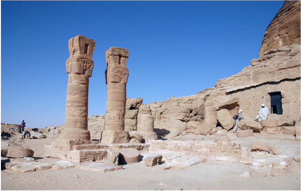
Fig. 37. The entrance to B 300, as it looked in 2010. The small white “talatat” blocks lying under the level of the standing columns belong to the foundations of the late 18th Dynasty temple called “B 300-sub.” They are now concealed by a modern mud brick pavement. (Photo: T. Kendall).
